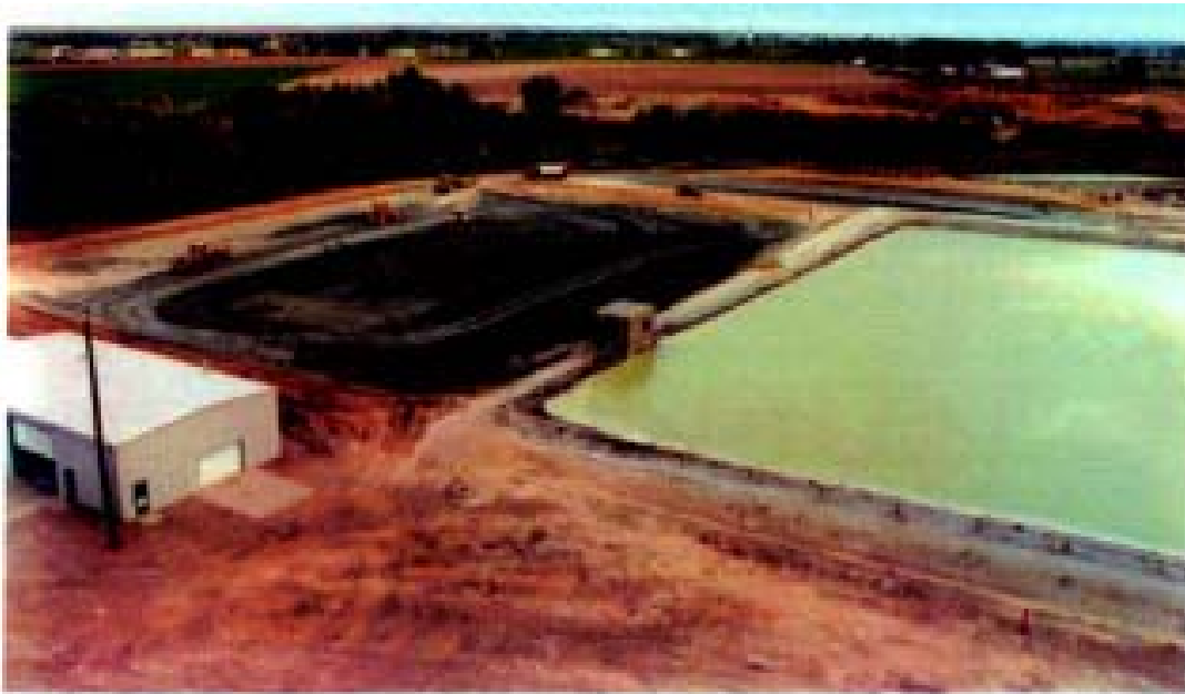
Photograph 2 – West Scrubber Pond Liner Construction
