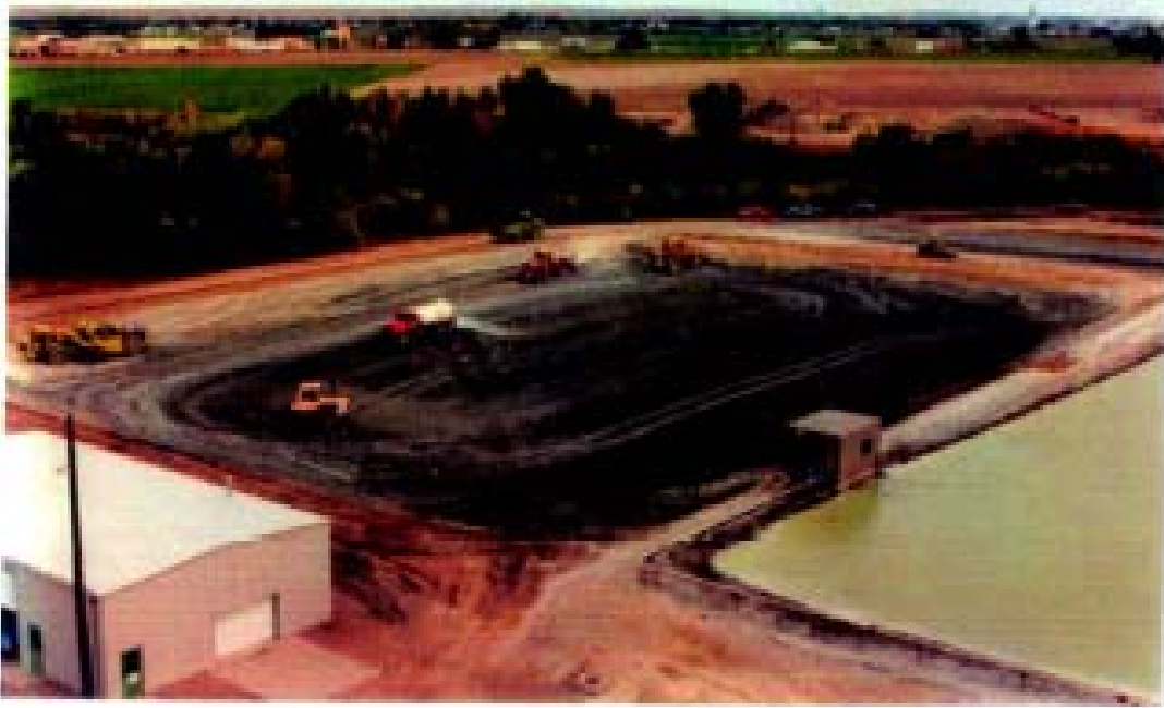
Photograph 1 – West Scrubber Pond Liner Construction
