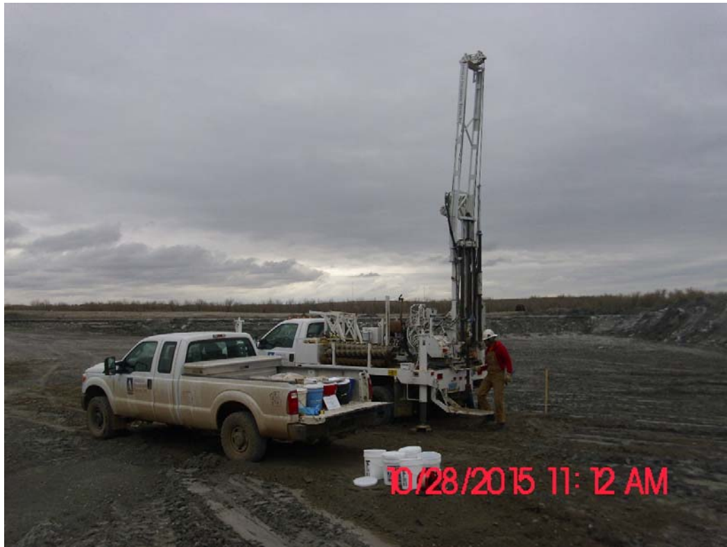
Photograph 5 – AET setting up to conduct drilling in the East Scrubber Pond
