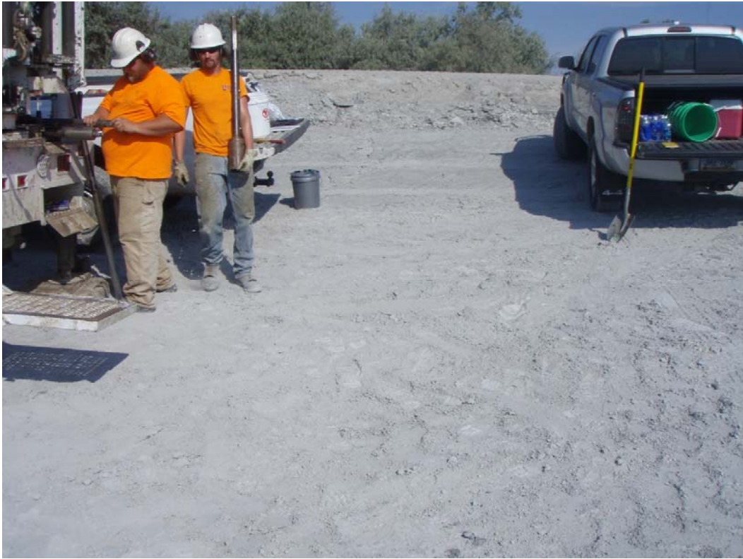
Photograph 1– AET setting up to conduct drilling in the West Scrubber Pond
